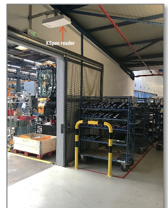
- Production area | logistics with xSpan RAIN RFID reader -
